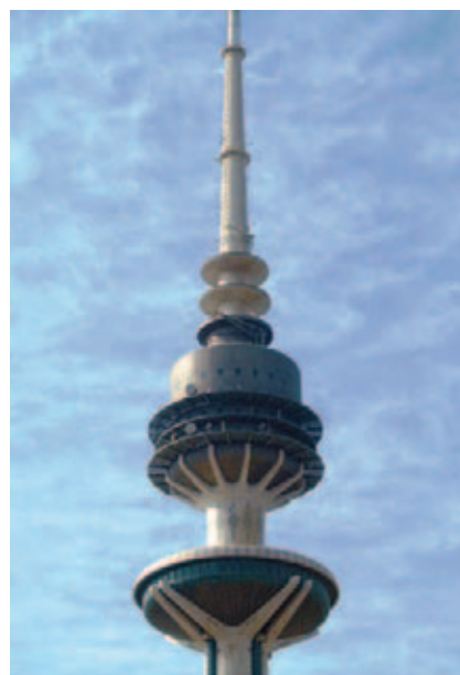
The 372-metre Kuwait Liberation Tower is home to the national telecom offices
