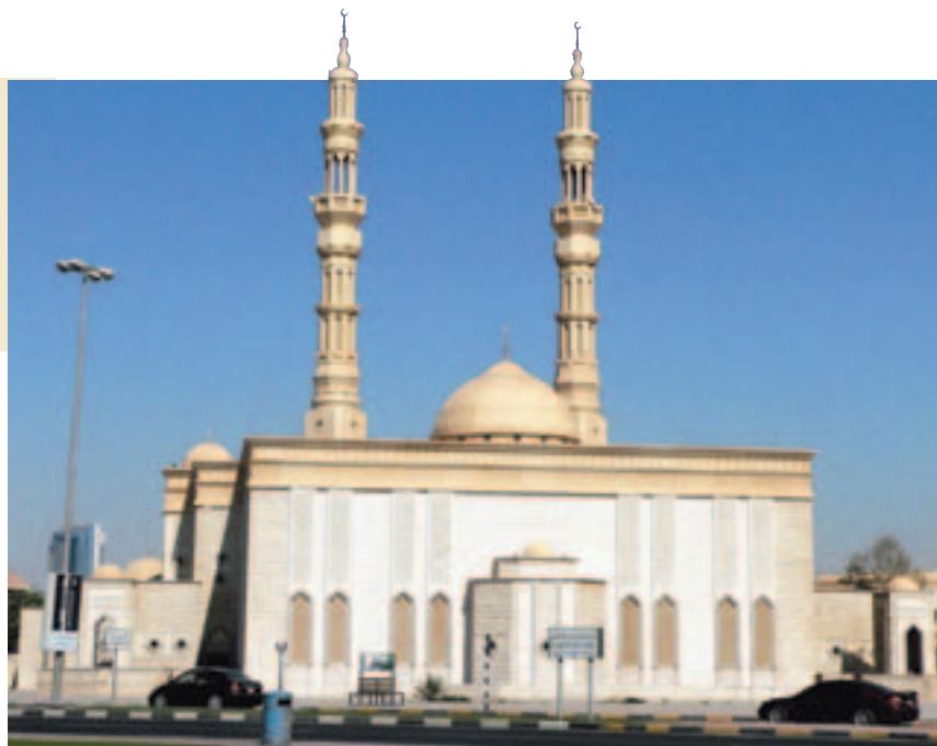
Traditional structures and stylish modern buildings vie for centre stage on Ajman's skyline
